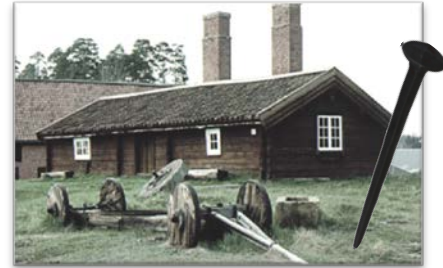
The house where the hammer-smithy was located in 1764
